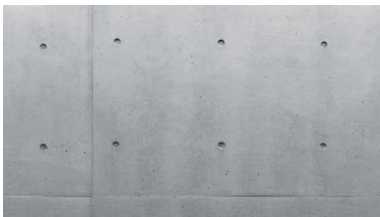
Concrete wall (with gypsum board substrate)
